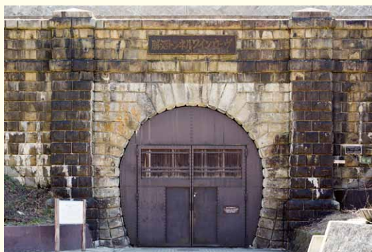
Of the tunnels in use when the Chuo Line opened, the former Fukazawa Tunnel is currently used as the "Katsunuma Tunnel Wine Curve." The 1,100 m long brick tunnel is valuable as a railroad culture heritage, and as a wine storage space, it provides an ideal environment for long-term wine maturation, with a year-round temperature ranging between 6 - 14 °C and humidity of 45% - 60%.
